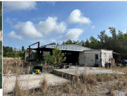
Rear view of house featuring a patio area
